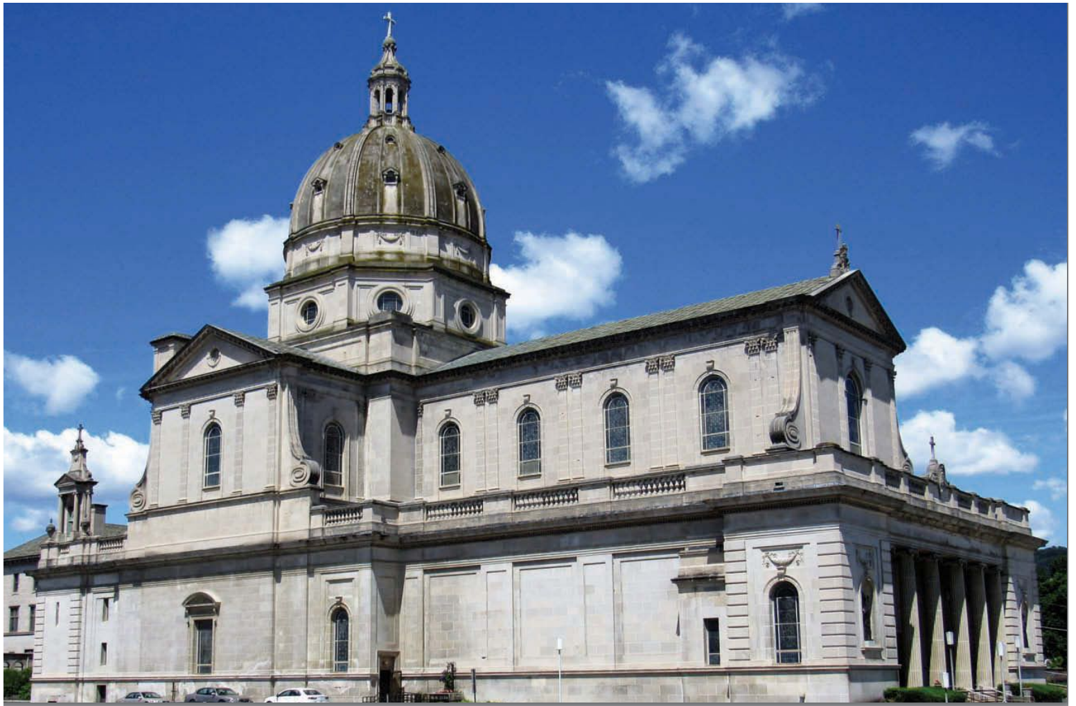
The Cathedral of the Blessed Sacrament, Altoona, Pennsylvania (photo: Farragutful)
